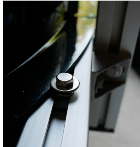
Figure 5 dome retaining bolts - help to keep the dome in the same place over time. Hand tighten only.
