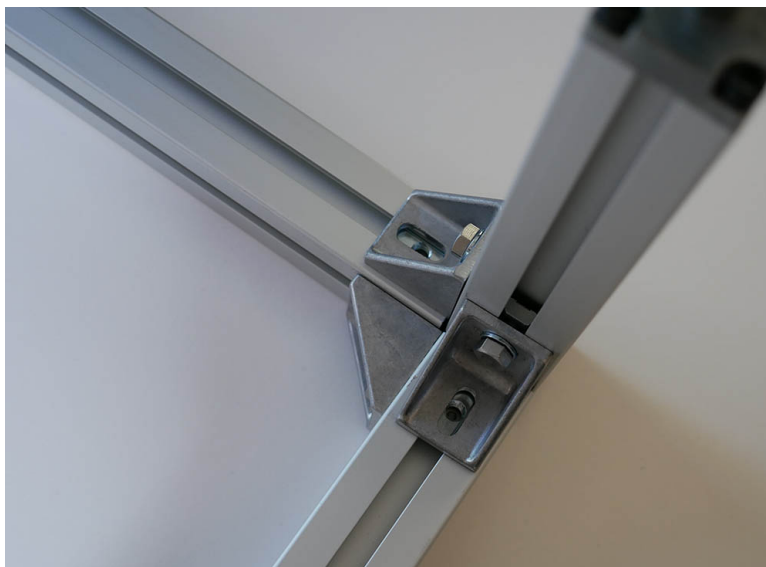
Figure 1 attaching the legs to the frame. Slide the nuts in to place first.
