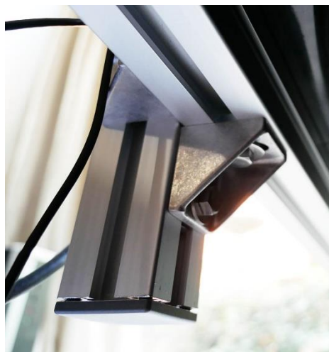
Figure 1 The vertical bars have some adjustment so you need to tighten a bolt when they are vertical. The third bracket underneath can be attached last when the top bar is levelled
